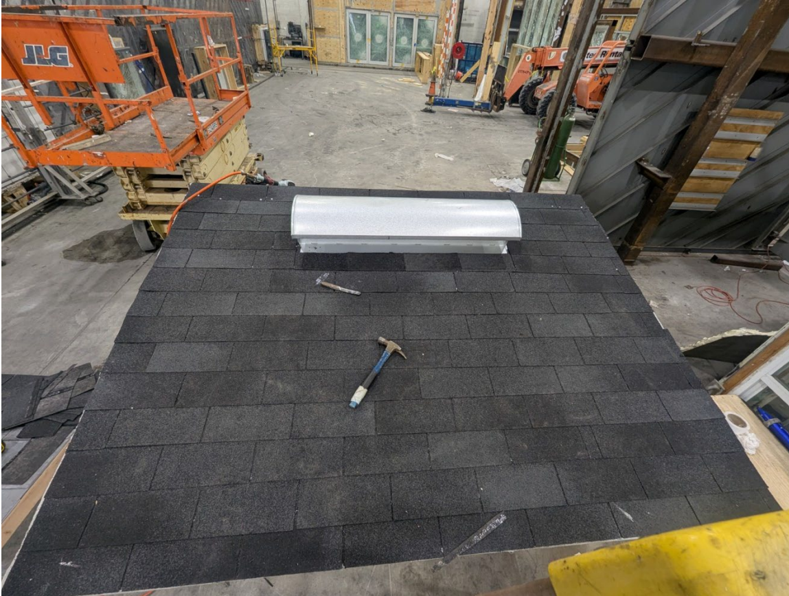
Photo No. 1 Top Side Before Testing
